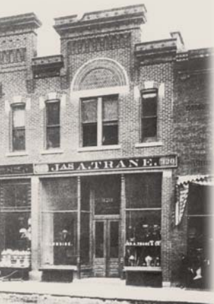
Trane Storefront La Crosse, Wisconsin 1891
